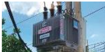
Amorphous transformers in power distribution, Yuko- Keiso, Vietnam
