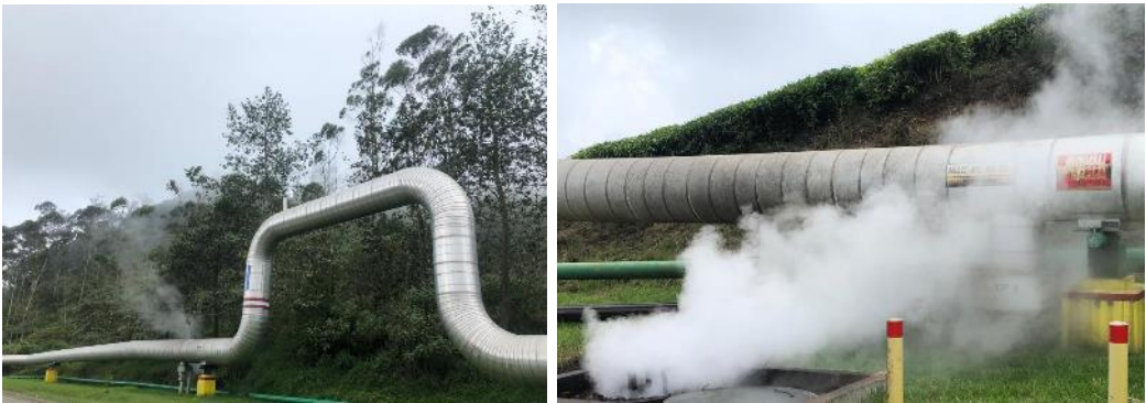
Geothermal steam pipes
