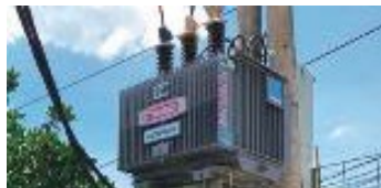
Amorphous transformers in power distribution, Yuko-Keiso, Vietnam
