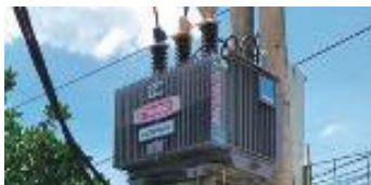
Amorphous transformers in power distribution, Yuko-Keiso, Vietnam
